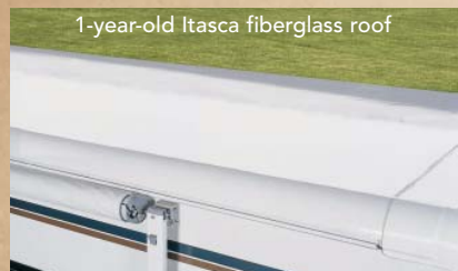
1-year-old Itasca fiberglass roof
