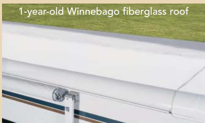
1-year-old Winnebago fiberglass roof
